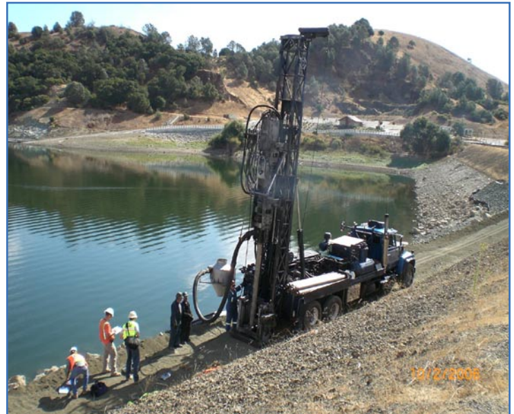
A drilling rig prepares holes for monitoring equipment at Anderson Dam.
