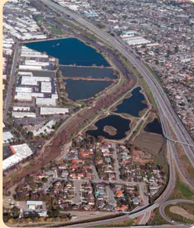
Groundwater recharge ponds (or percolation ponds) adjacent to Los Gatos Creek and Highway 17. These ponds are kept filled with water from Lexington Reservoir or imported water from the Delta.
